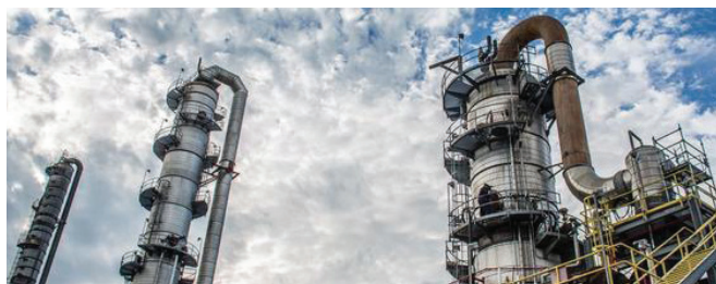
Ascend Performance Materials' Decatur facility is one of only four plants in the world that produce ADN on a large scale. (Photo courtesy of Ascend Performance Materials)
